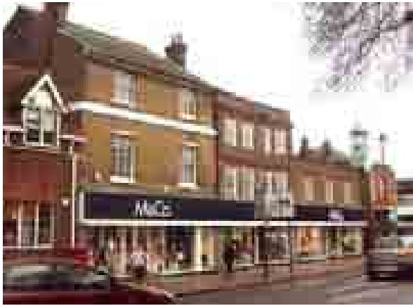
Extended shopfronts at 220 - 212 High Street with bold lettering to the fascia
