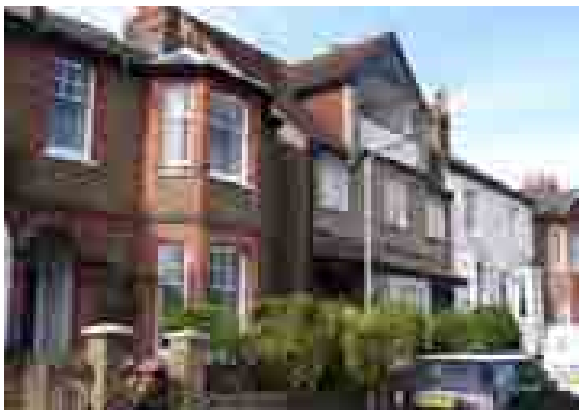
Nos.17 to 25 Charles Street
