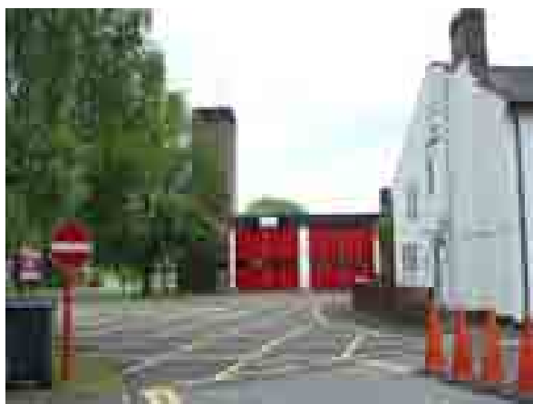
Fire and Ambulance Station, Castle Street
