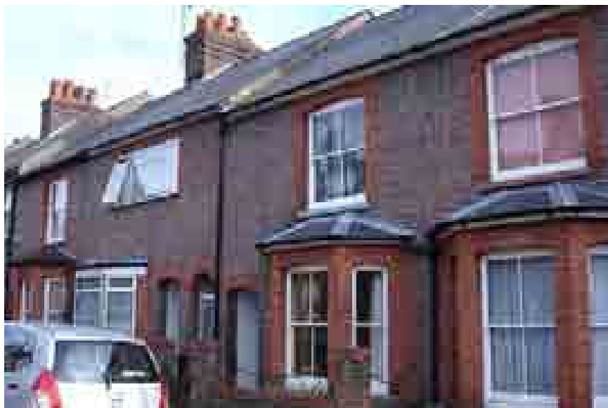
Terrace on Clarence Road showing typical materials (and poor replacement windows to middle left)
