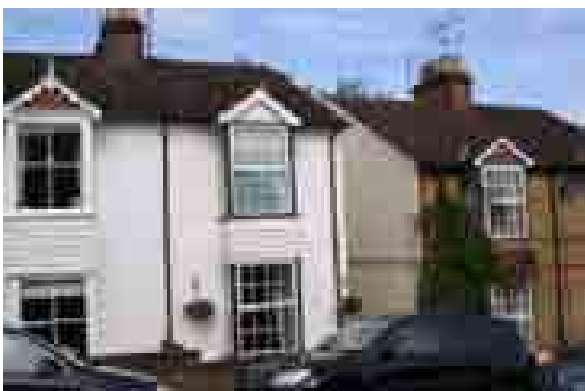
A concentration of inappropriate replacement windows at Kitsbury Road
