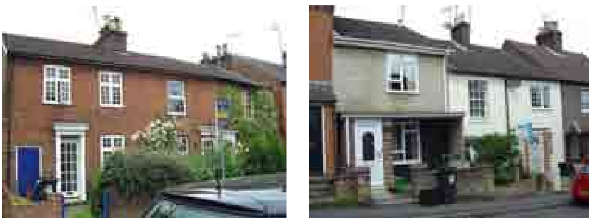
Replaced doors, windows and slate roofs on Holliday Street and Victoria Road
