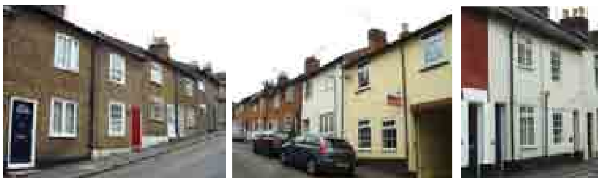
Replaced doors, windows and slate roofs on Highfield Road and Ravens Lane
