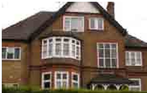
Poor alterations at 13 Shrublands Road
