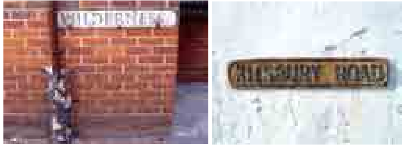
Road name signs which need some general maintenance
