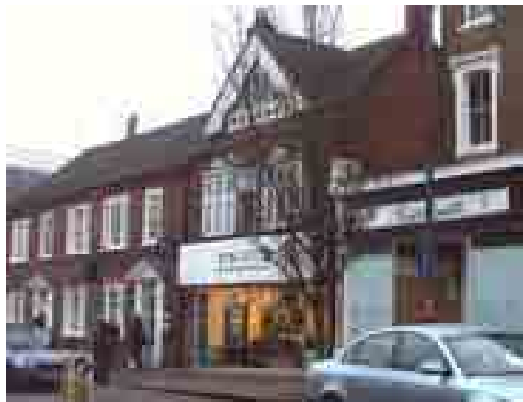
Inserted modern shopfront into an older property at 193 High Street next to a listed building
