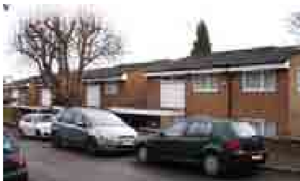
Langdale to Mooring at the south end of Doctor's Commons Road
