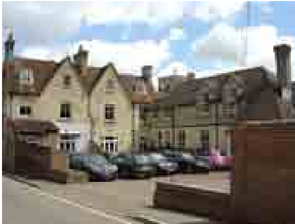
137 High Street: rear plots now with parking (Chesham Road)
