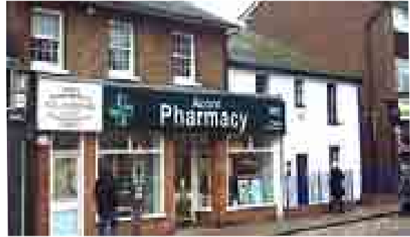
256 High Street (Acorn pharmacy) built-out on the ground floor with bold signage
