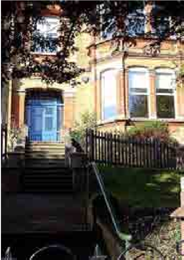
Stone door and window arches
