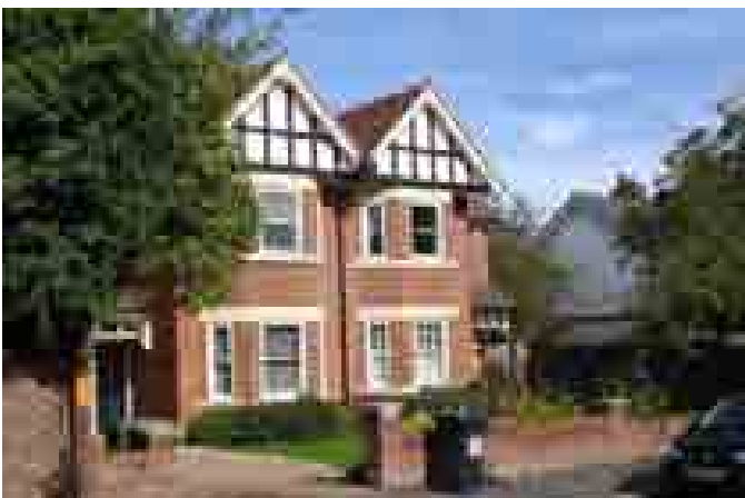
New houses at 20 Montague Road
