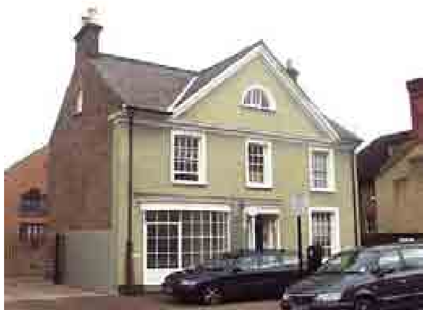
108 High Street, The Dower House (High Street Central)
