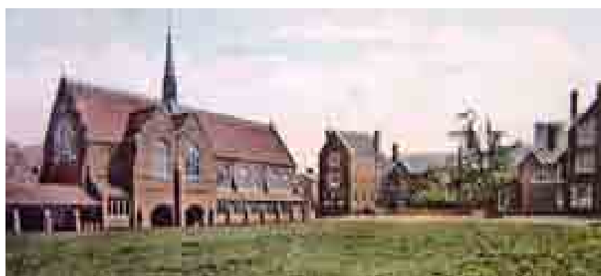
Berkhamsted School from inside the quad c1904 showing the new chapel and Old Hall (HALS Photographic Collection)
