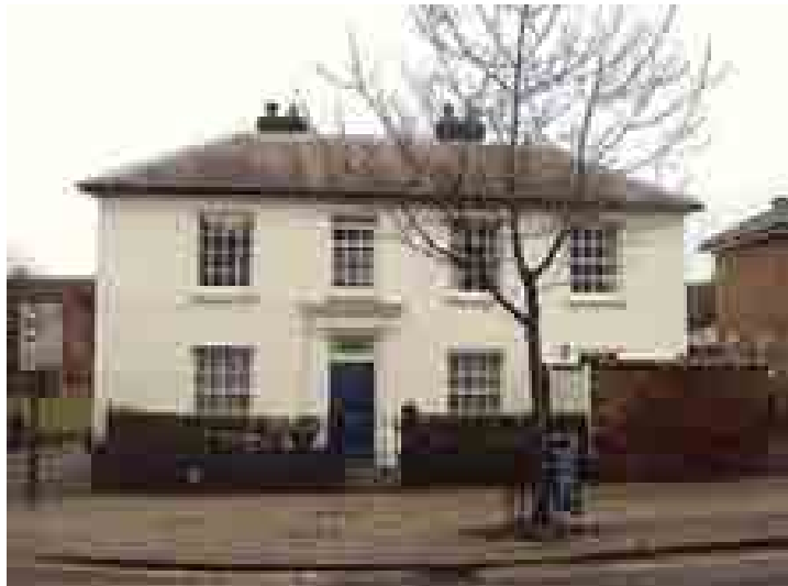
120 High Street with its original front boundary
