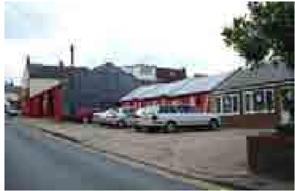
Workshop and offices on Park Street (behind 352 High Street)
