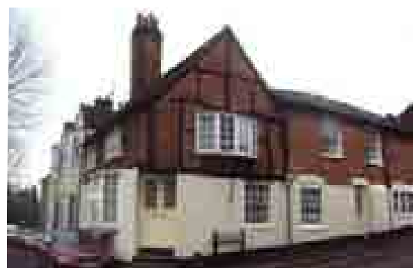
51 & 53 High Street (High Street East)
