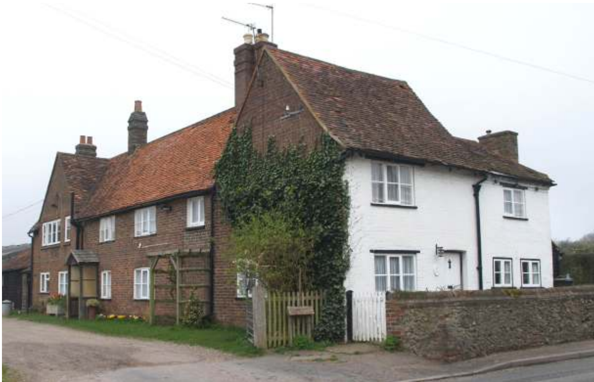
Tuffs Farm, a timber-framed building cased in brickwork
