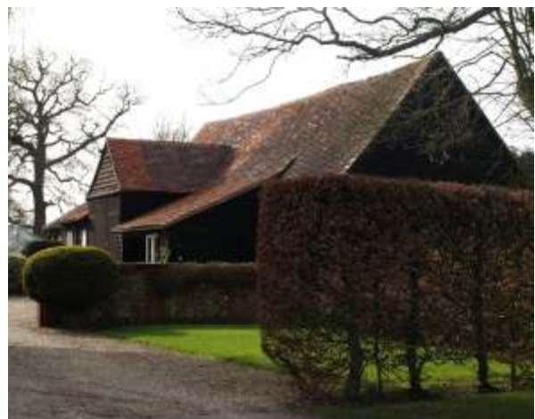
The Barn at Braziers Farm is a listed building
