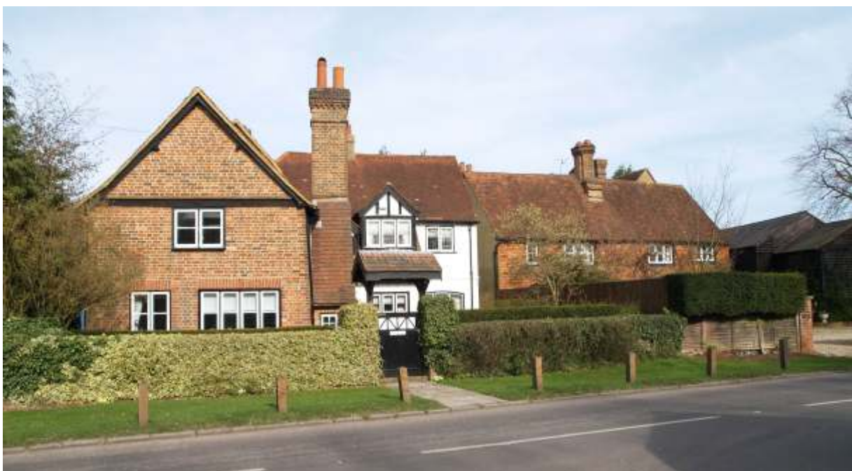
Tiled roofing predominates in the Conservation Area. Notice the plain mortared verge to the gable end. Also the tiled offset to the chimney and tiled canopy to entrance gate. The Tile House to the right, was re-modelled in the early C20th, when the tile-hanging, which obscures the original framing, was introduced
