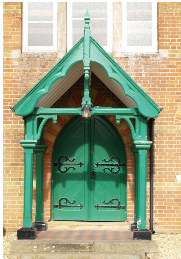
The Baptist Chapel, a locally listed building
