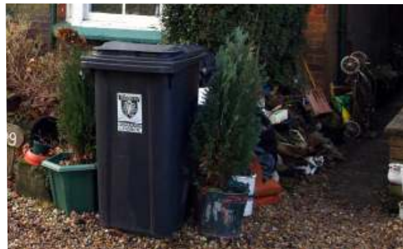
The appearance of these houses is spoilt by external visual clutter, as well as by unfortunate changes to the fenestration so that the original symmetry has been upset
