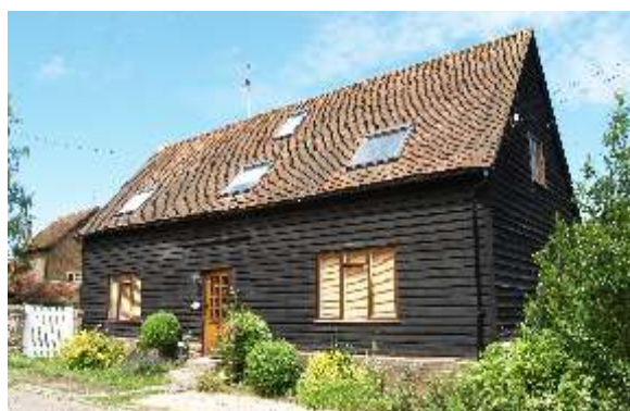
Residential conversion with prominent rooflights, aerial, external lighting etc.
