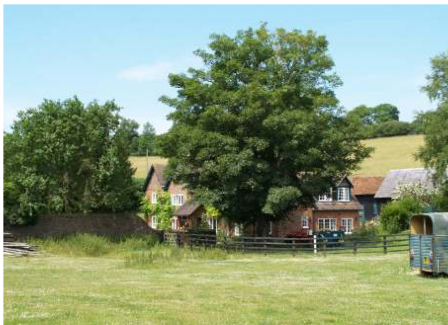
Buildings in Frithsden Conservation Area are characterized by their modest scale, and unobtrusive siting
