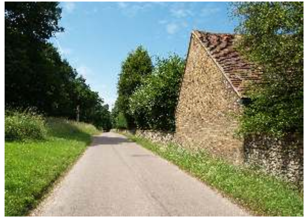
Looking west along the valley bottom, with Frithsden Copse on the left. The extended flint wall reinforces the strong linear nature of the settlement. The managed woodland, wall, yellow brickwork etc. all demonstrate the impact of the Ashridge estate on the Conservation Area.
