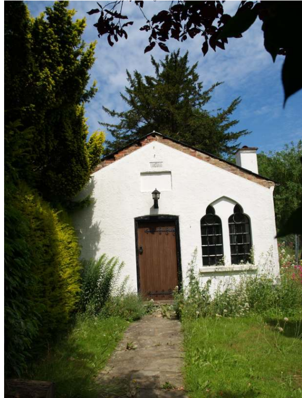
The Bethesda Chapel – a locally listed building
