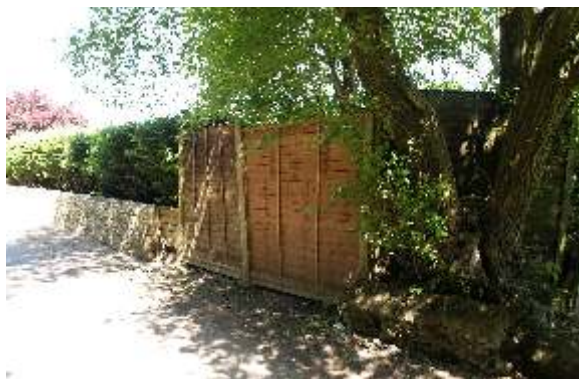
Inappropriate boundary treatment
