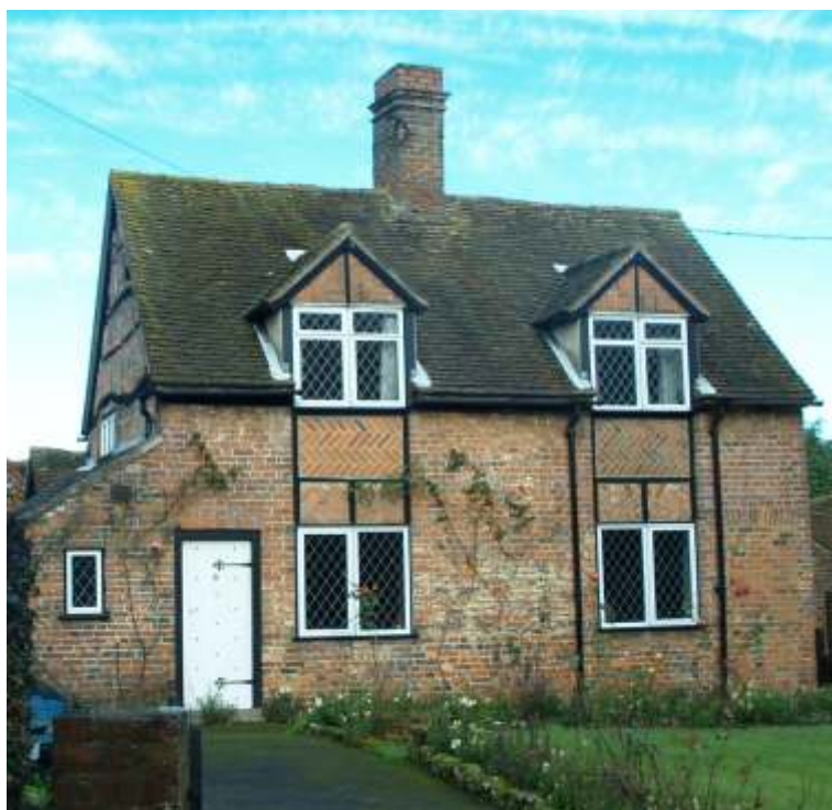
Adjacent to The Glebe House, these former pair of semi-detached cottages are probably late C17th with light timber-framing and brick infill. The dormers and herringbone brickwork are C20th insertions
