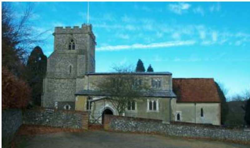
Church of St John the Baptist – flint, stone, brick, render, clay peg tiles and lead
