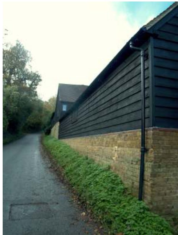
The converted farm buildings at Church Farm turn their back on Piper's Hill
