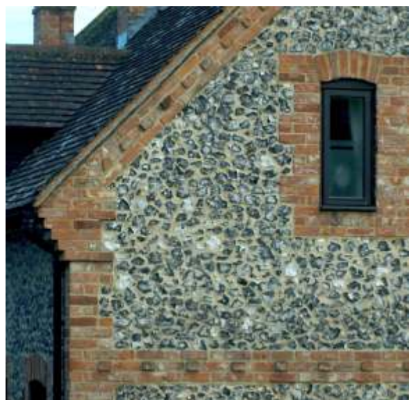
C20th brick and flint detailing to Church Farm Cottages
