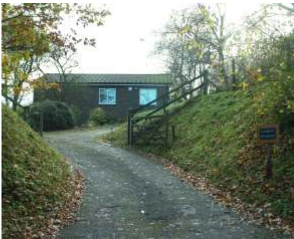
Buildings on the south side of Pipers Hill such as the Vicarage weaken the character of the Conservation Area
