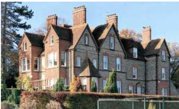
The Old Vicarage, Pipers Hill. C19th flint and brick – note the clusters of octagonal shafts to the chimney stacks
