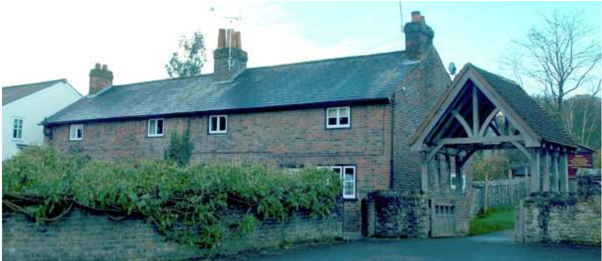
Darker plum brickwork to Nos. 5, 6 & 7 Church Cottages
