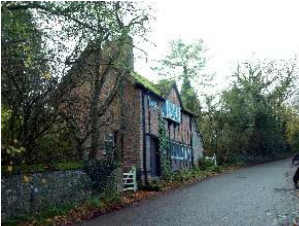
1, Pipers Hill is a listed building, its condition a cause of concern at time of survey
