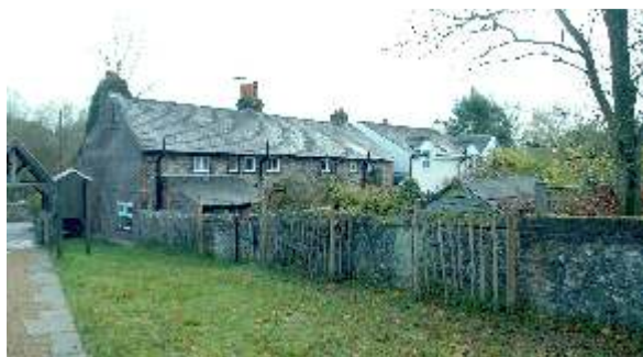
Flint used in the rear wall of Nos 5, 6 & 7 Church Cottages and in the boundary wall of the Churchyard. Note also slate used for flatter pitched roofs
