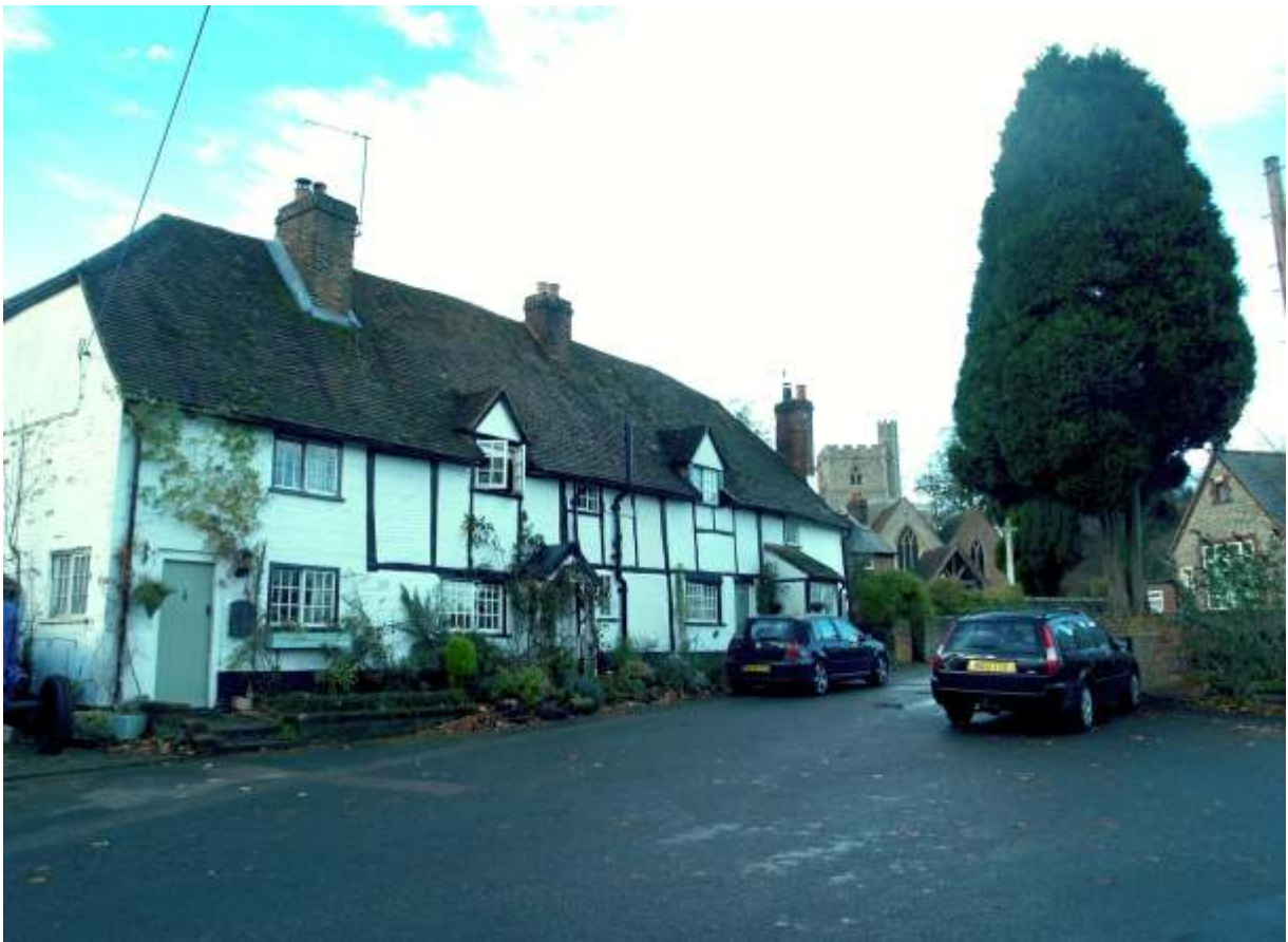
View of the Church flanked by Church Cottages and School
