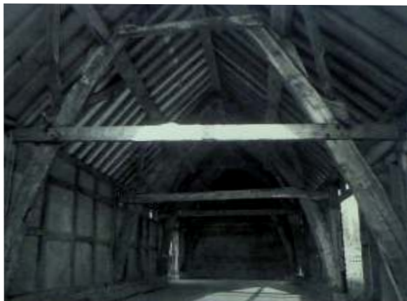
Interior of Cruck Barn 1994 (Hastie)
