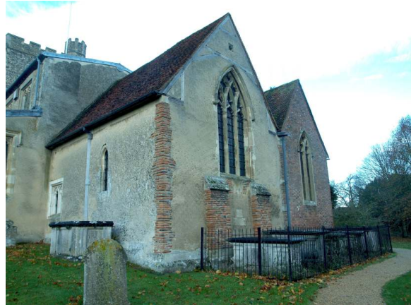
Roman bricks re-used in the East end wall of Great Gaddesden Church
