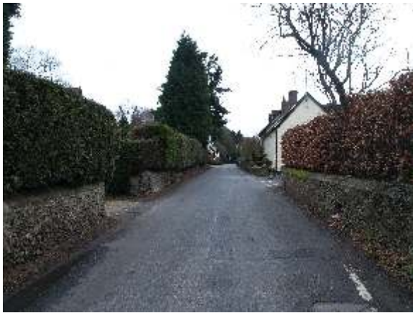
Flint used in boundary walls
