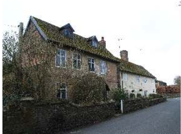
Timber frame, brick (both limewashed and unpainted) clay tile roofing and flint boundary wall
