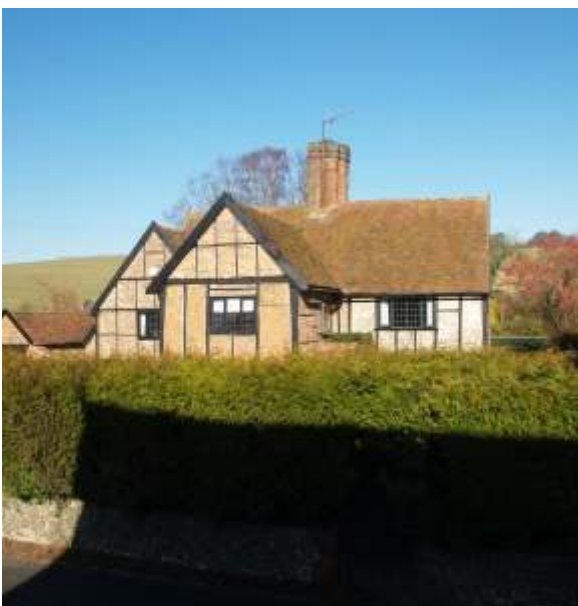
Chimney at Pipers Forge
