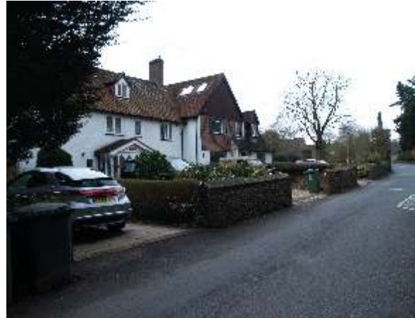
The rooflights are prominently sited, and break up the otherwise uninterrupted, plain roofs which are a characteristic feature of the Conservation Area
