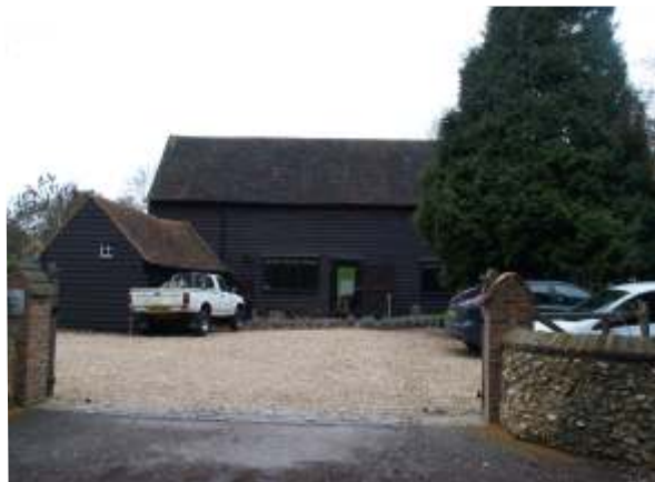
Further conversion of ancillary buildings in Nettleden should be avoided
