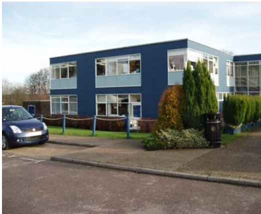
Photo 1: Main school building
