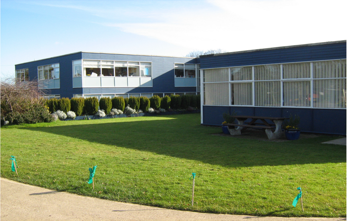
Photo 1 View of the Main School Building
