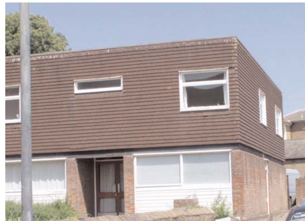
The siding and flat roof do not work within local styles.
