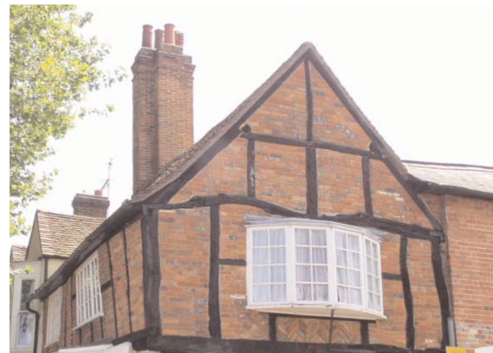
This High Street listed building has timber framing infilled with brick.
