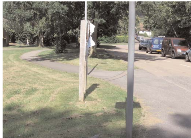
The pavement leaves the side of the street, creating a rustic feel to the area.
