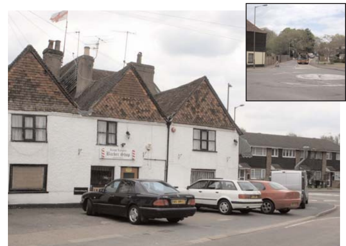
This listed building could serve as a useful gateway to the canal towpath.
