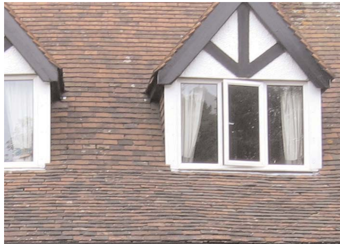
This residential building shows a red clay tiled roof with a modern application of Tudor-style timber framing.
