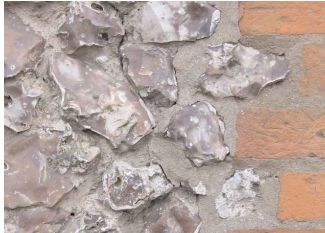
Knapped flint with brickwork forms one of the most distinctive styles applied in Kings Langley. As can be seen in the image above, the flint is not squared. The flint has been cut roughly, producing a rustic quality. (Located on west side of the High Street)
