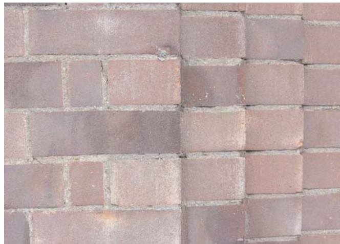
Brick is the predominant material in Kings Langley, and the village is marked by a tremendous variation in its application. In this instance where two buildings meet on The Nap, one wall shows an alternation between headers and regularly placed bricks while the other wall shows a consistent application of headers.
