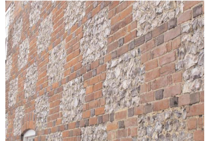
In a few instances within the vicinity of the village centre, buildings employ both knapped flint and brickwork. In this particular building, the old brewery on Church Lane, the brickwork alternates between blue headers (known as 'clinkers') and standard bricking.
