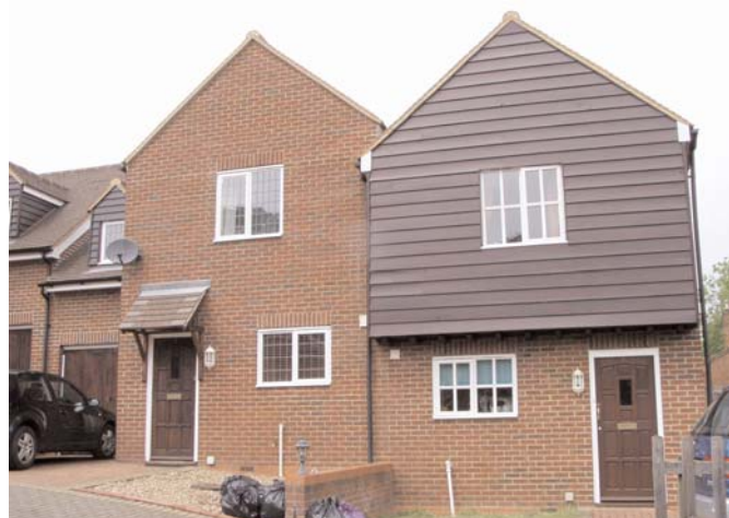
The newer buildings in Kings Langley tend to be built with machine-made brick, and frequently incorporate other materials as well. These particular homes off the High Street employ less traditional wood cladding.
