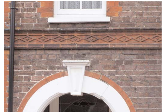
In addition to the elaborate brickwork, this Victorian building exhibits a rounded arch with a decorative voussoir (keystone).
