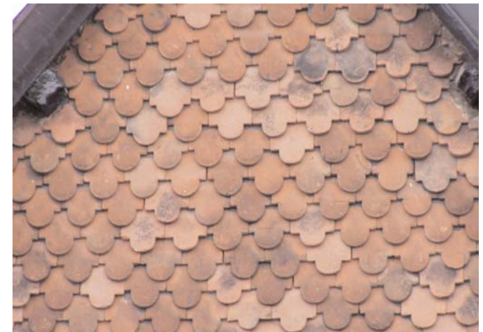
This High Street building provides an example of scalloped terracotta tiling.
