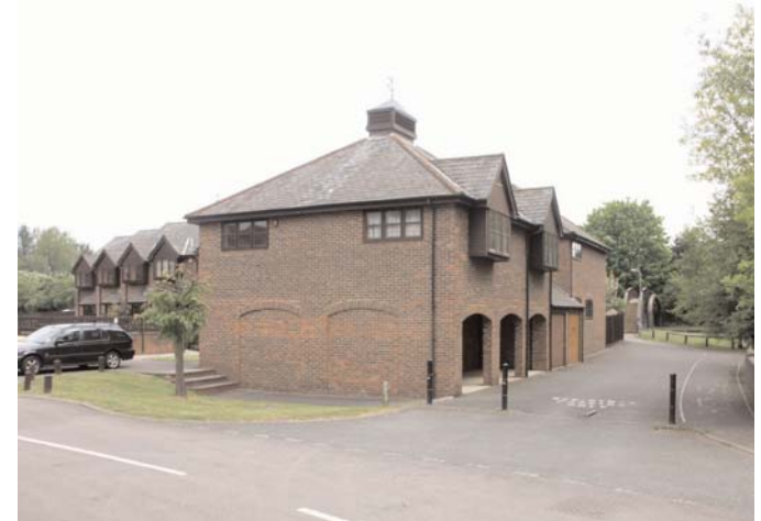
These gabled houses on the site of the old Corn Mill on Mill Lane use machine-made brick. The application of a weathervaned top and mock arches are nods toward traditional design. The Mill Lane area is also distinguished by a considerable degree of asphalt paving including the path to the Canal Walk.
