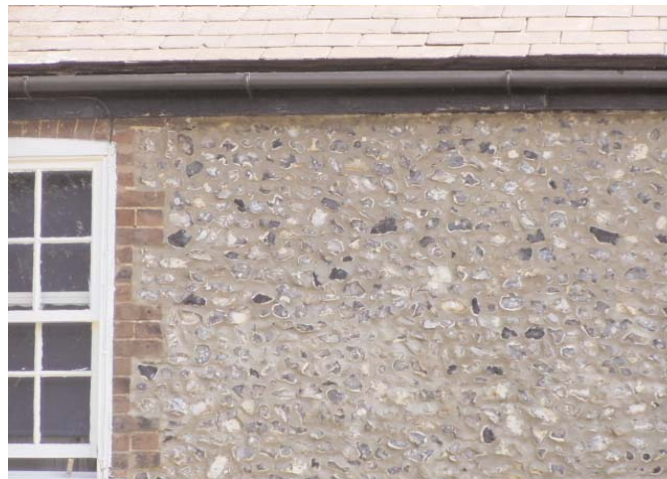
Flint is the principal indigenous building stone, although chalk lump can sometimes be found in the area. Welsh slates were imported after the opening of the canals and railways.
