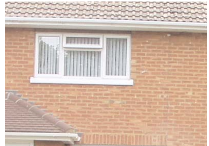
The image above is an example of a modern building with a clay tile roof and machine-made bricks. Consultation participants were concerned with the quality of many modern buildings.
