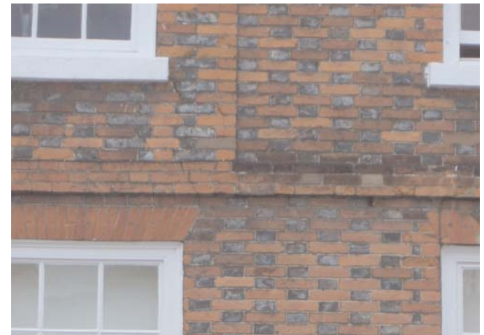
Diaper brickwork using blue 'headers' and red 'stretchers' was a common decorative motif in the 19th century.
