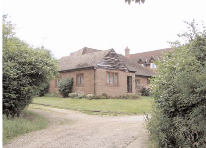
1. Detached house with private driveway and front and rear gardens: Grange Close
