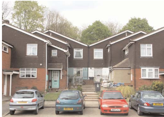
3. Staggered terraced housing with small or no front garden, no on-site parking and a private rear garden: Roman Way.
