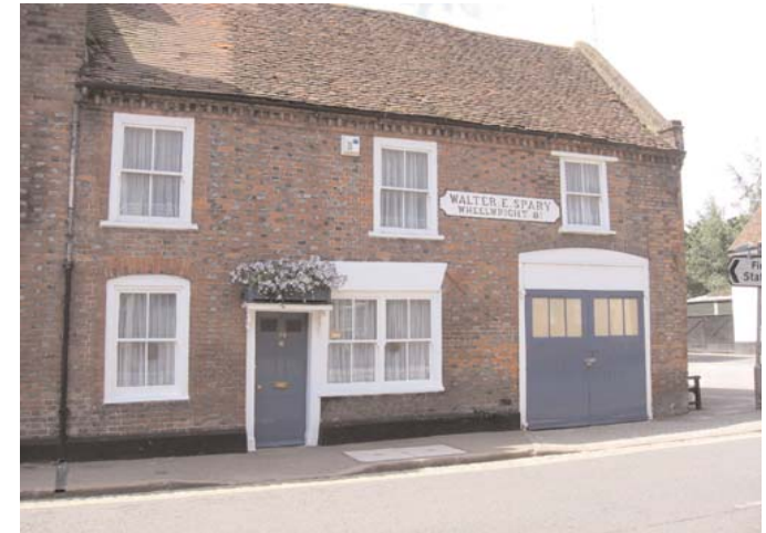
Cottage c. 1850. Until the 20th century building materials were sourced locally: red and blue bricks and handmade plain clay tiles.
