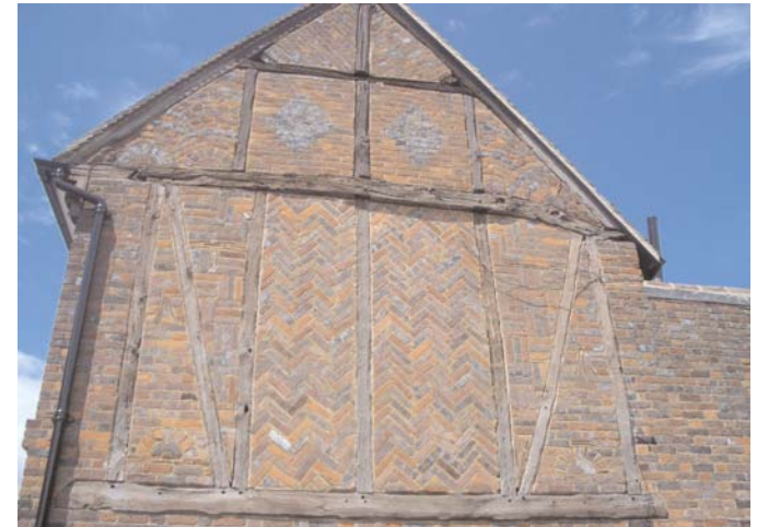
The timber framed tradition shown above is infilled with bricks, often used to replace former plaster panels.
