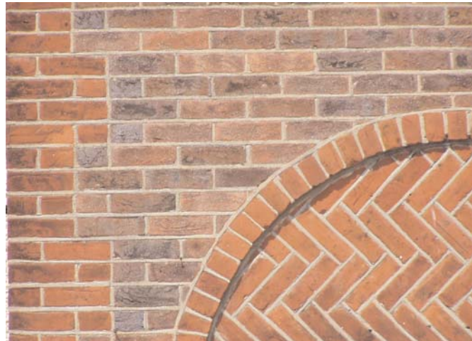
This image shows high quality modern brick detailing.
