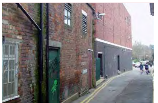
Older buildings and electricity substation next to the existing Tesco store
