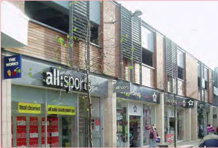
Recent development in Boston, Lincolnshire that successfully integrates upper storey car parking into the elevations
