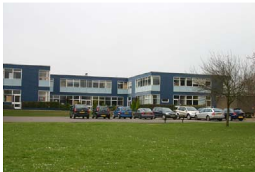
Existing school buildings
