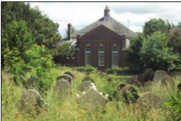
Baptist Chapel, Akeman Street, west elevation and graveyard
