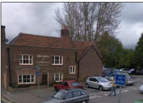
31 Frogmore Street, front (south) elevation
