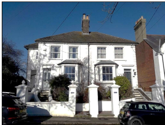
Original boundary walls and piers at Lynwood and Farleigh on Park Road
