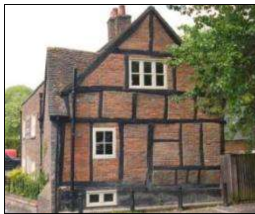
31 Frogmore Street, exposed timber framing and brick-nogging to the east elevation
