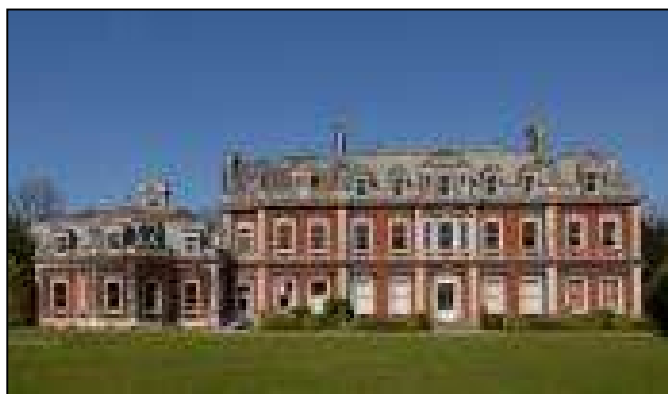
Tring Park Mansion (Grade II*)
