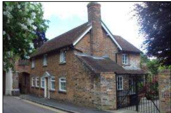
uPVC windows in Vicarage Lodge, Churchyard
