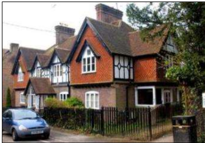
5, 6 and 7 Park Street. Typical use of 'Rothschild' materials including brick, decorative timber framing and tile-hanging
