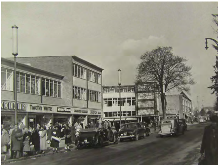
Figure 22: Images of Hemel Hempstead New Town shortly after construction. The pool and fountain (top) stood opposite the entrance to Bank Court (DBC Archive)
