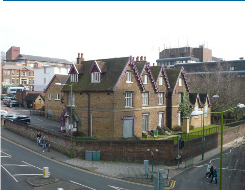
Figure 30: Cheere House, presently boarded and with no future use identified
