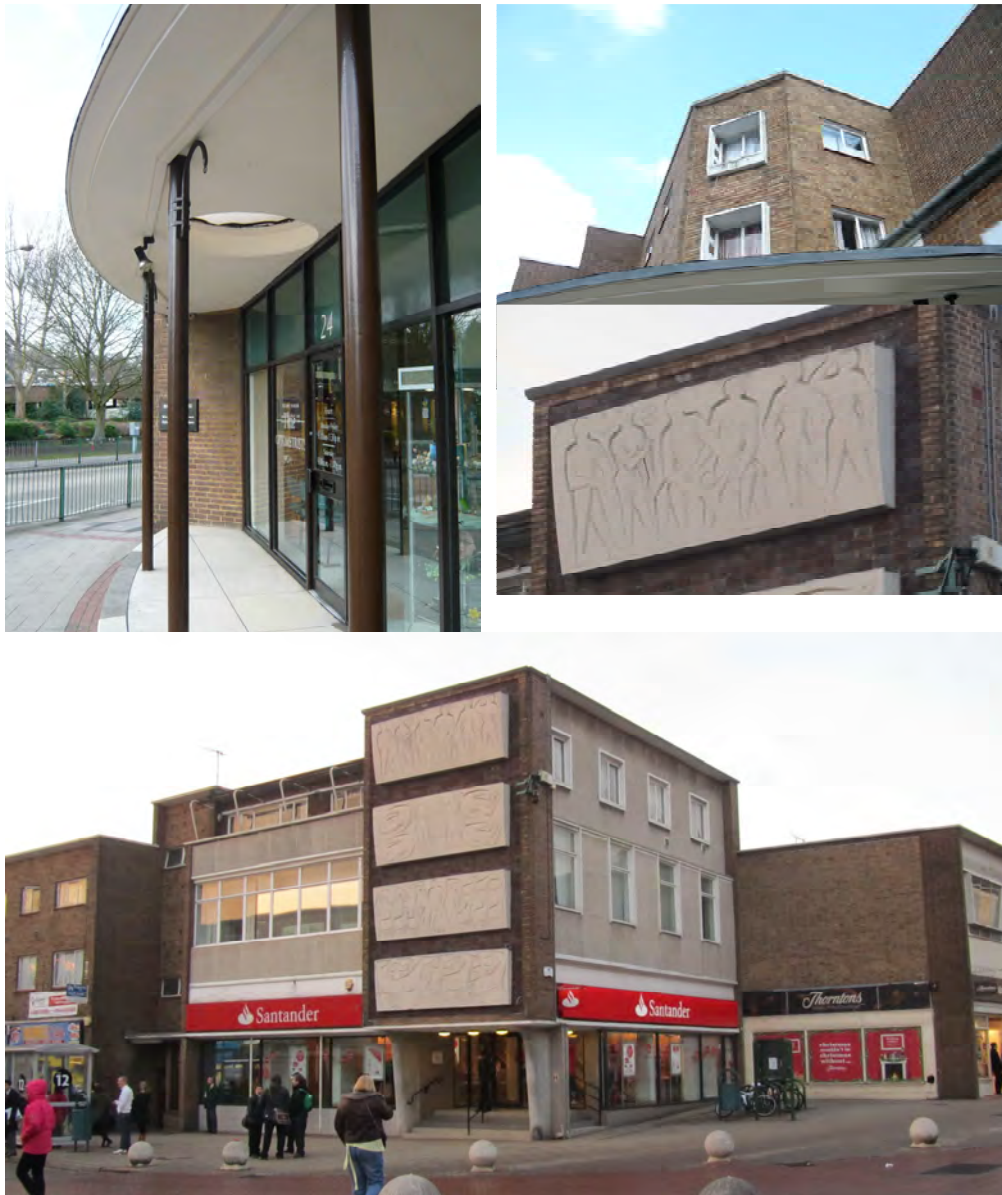
Figure 24: Architectural detailing to buildings in Bridge Street
