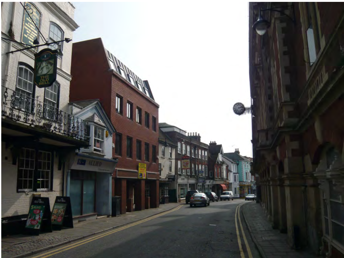
Figure 12: 45-47 High Street - Simple improvements to this building such as the painting of the brickwork would improve its appearance of this building.
