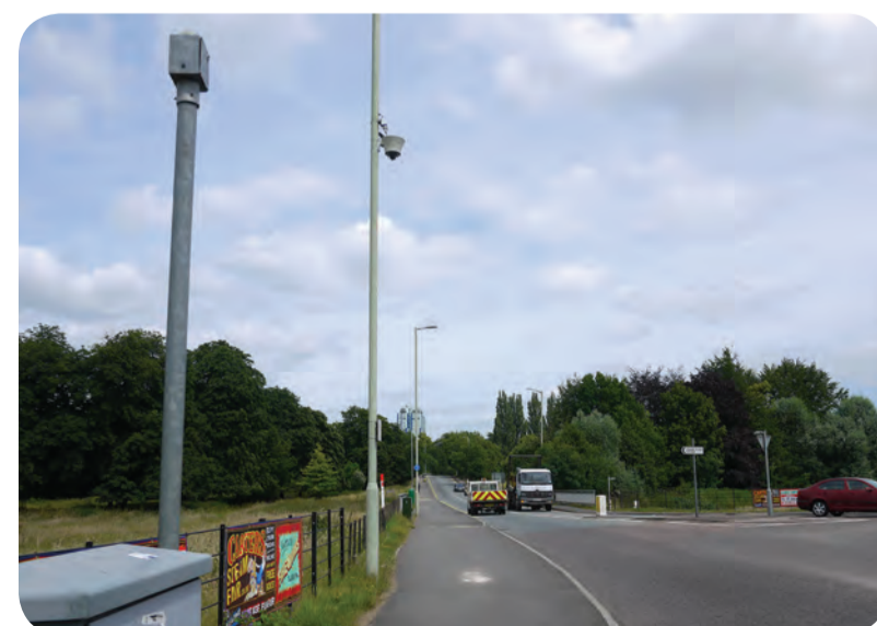
London Road and Station Road Junction
