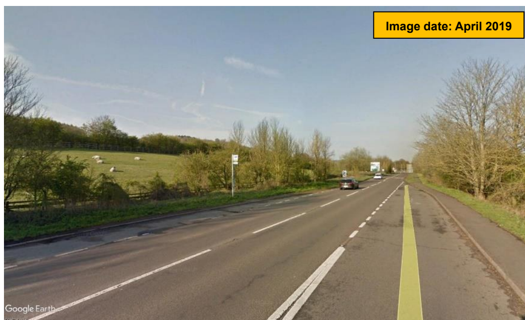
Figure 5-24: Narrow footway on one side of the road and no footway or crossing at the bus stop on London Road
