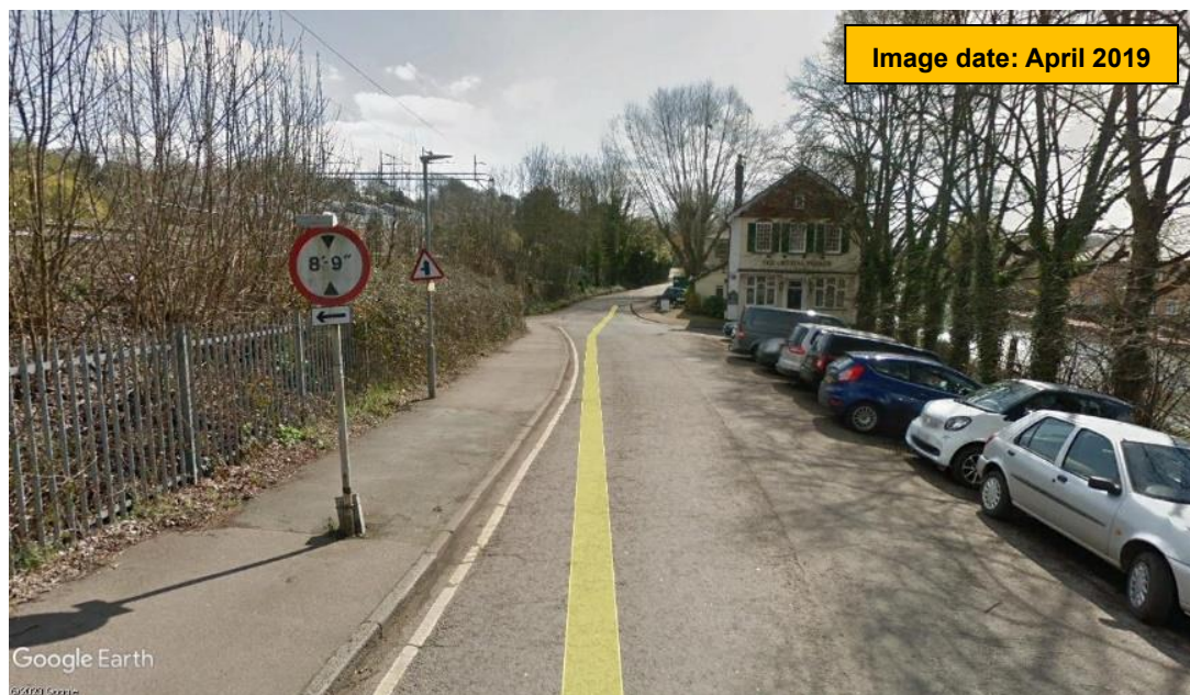
Figure 5-4: Road signs on footway on Station Road
