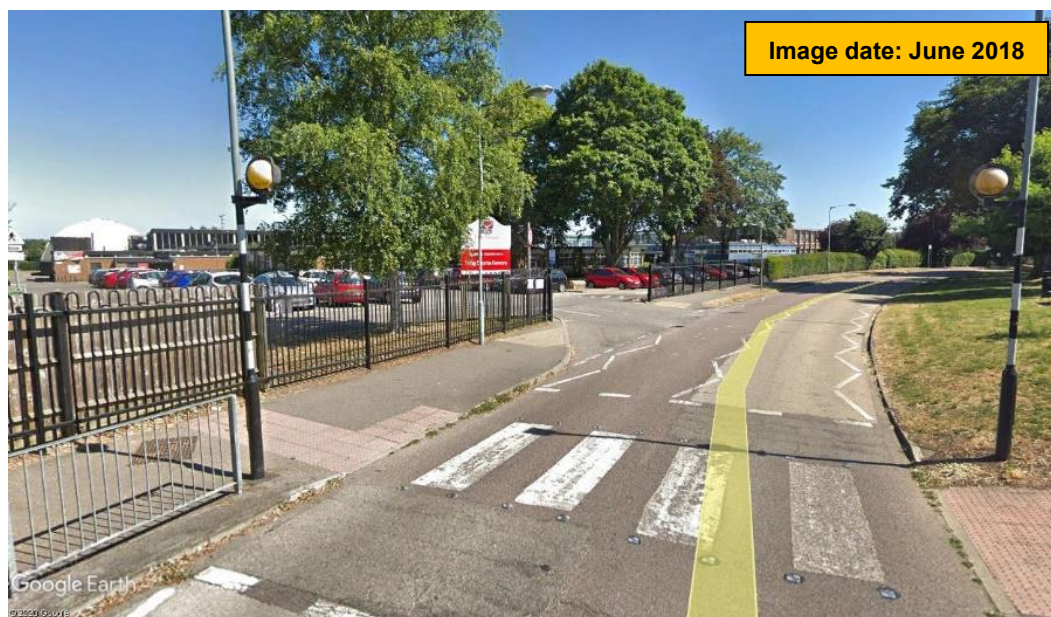
Figure 5-23: Faded markings on zebra crossing outside Tring School
