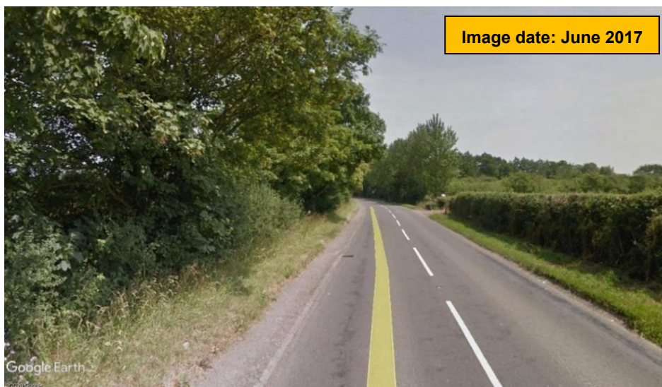
Figure 5-26: Highway verge encroaching onto footway on Bulbourne Road
