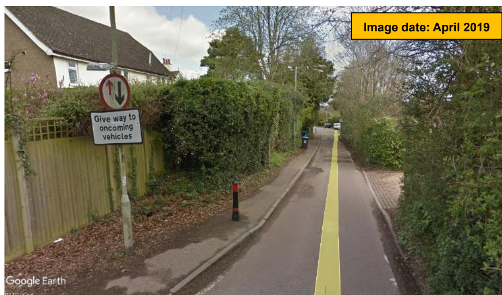
Figure 5-14: Signage and bollards obstructing the footway on Cross Oak Road
