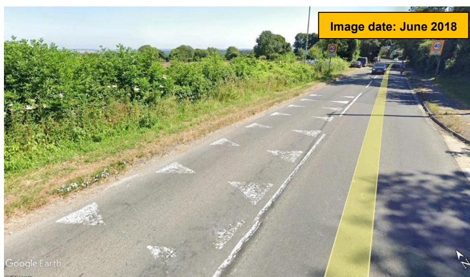
Figure 5-21: Faded dragon's teeth on Icknield Way to reduce speed to 40mph outside Icknield Way Industrial Estate
