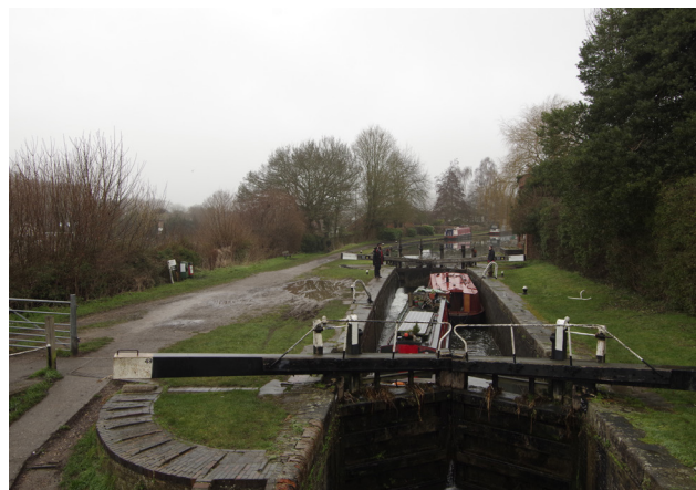
View of south-western boundary facing north-west along Grand Union Canal towpath
