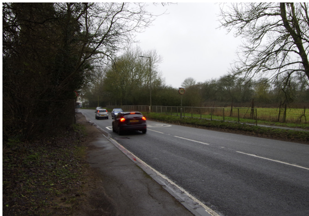
View taken from north looking along north site boundary.
