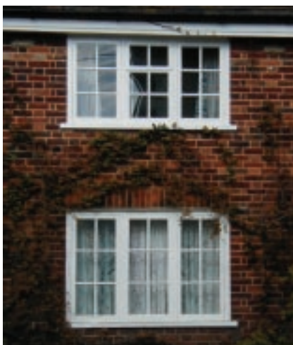
Well proportioned & positioned glazing bars
