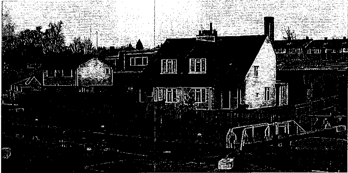
The existing Lock House, Apsley Lock
