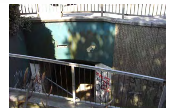
Underpass entrance at Heath Park Gardens
