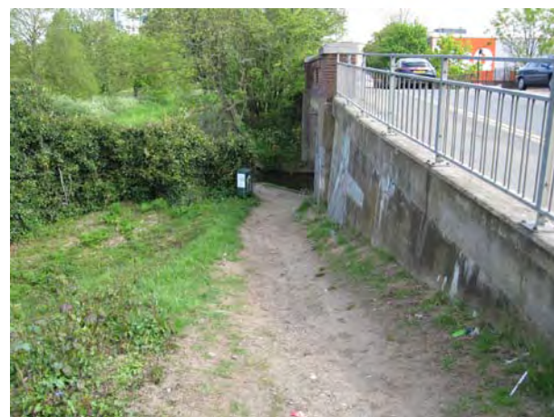
Existing view looking north showing an informal descent to the Grand Union Canal adjacent to the bridge crossing the canal at Two Waters Road.
