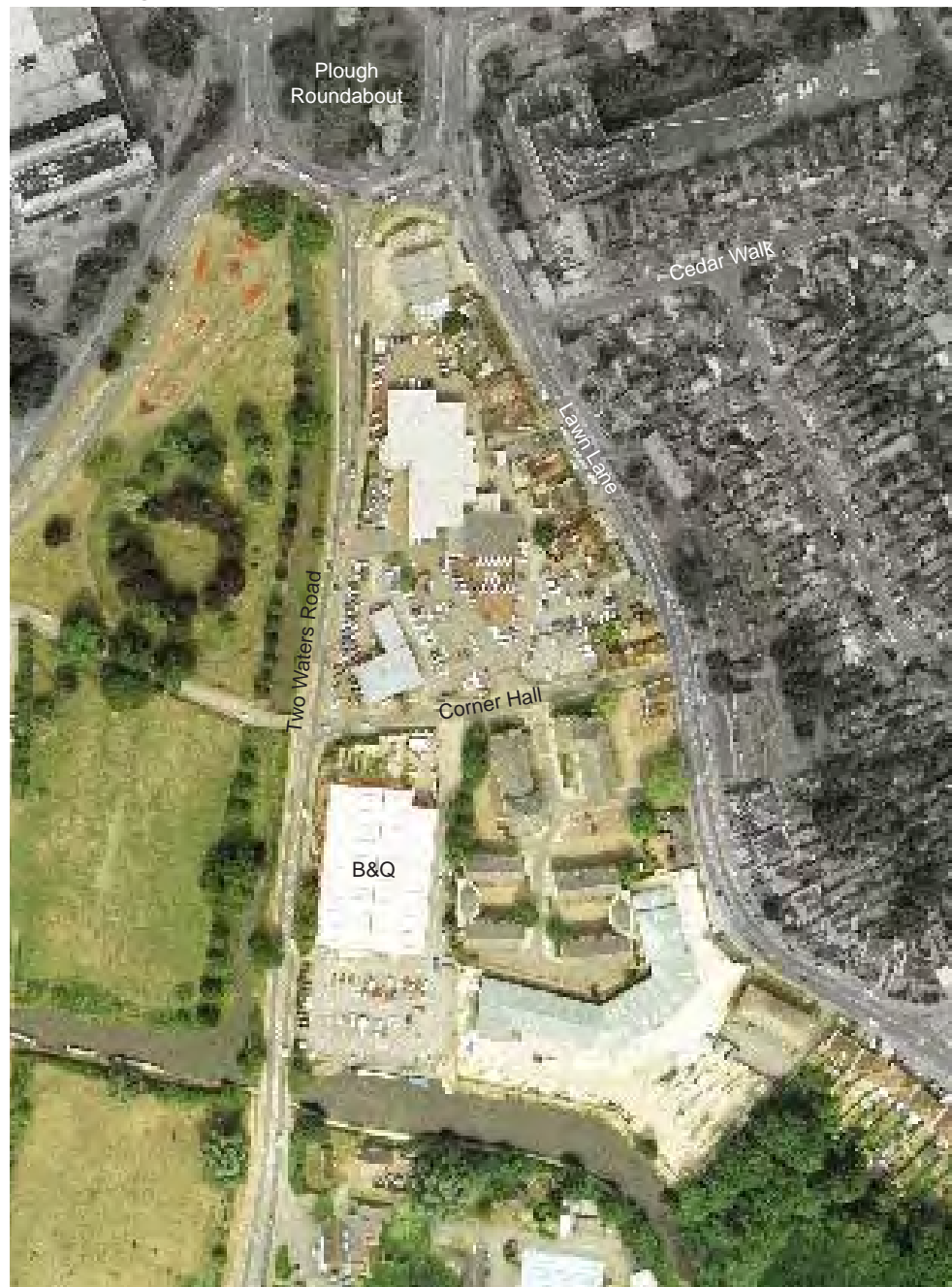
Aerial view of existing site
