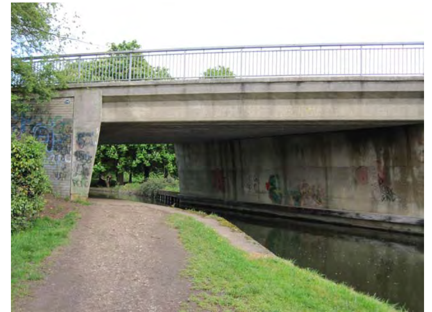
Existing view east along the towpath showing the road bridge across the Grand Union Canal at Station Road.
