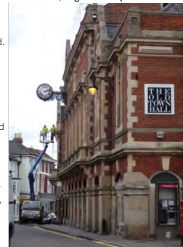
Old Town Hall, High Street (Source : DBC)
