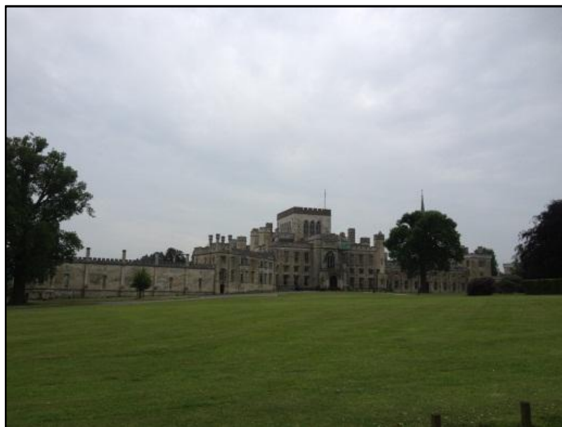
View to Ashridge House located within open Green Belt setting
