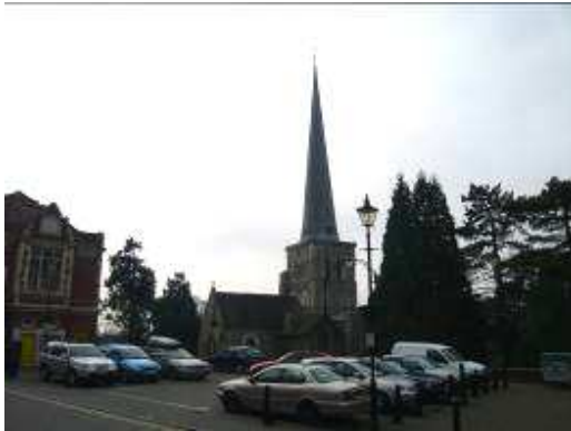
Figure 7: The dramatic impact of the spire in views from St Marys Close
