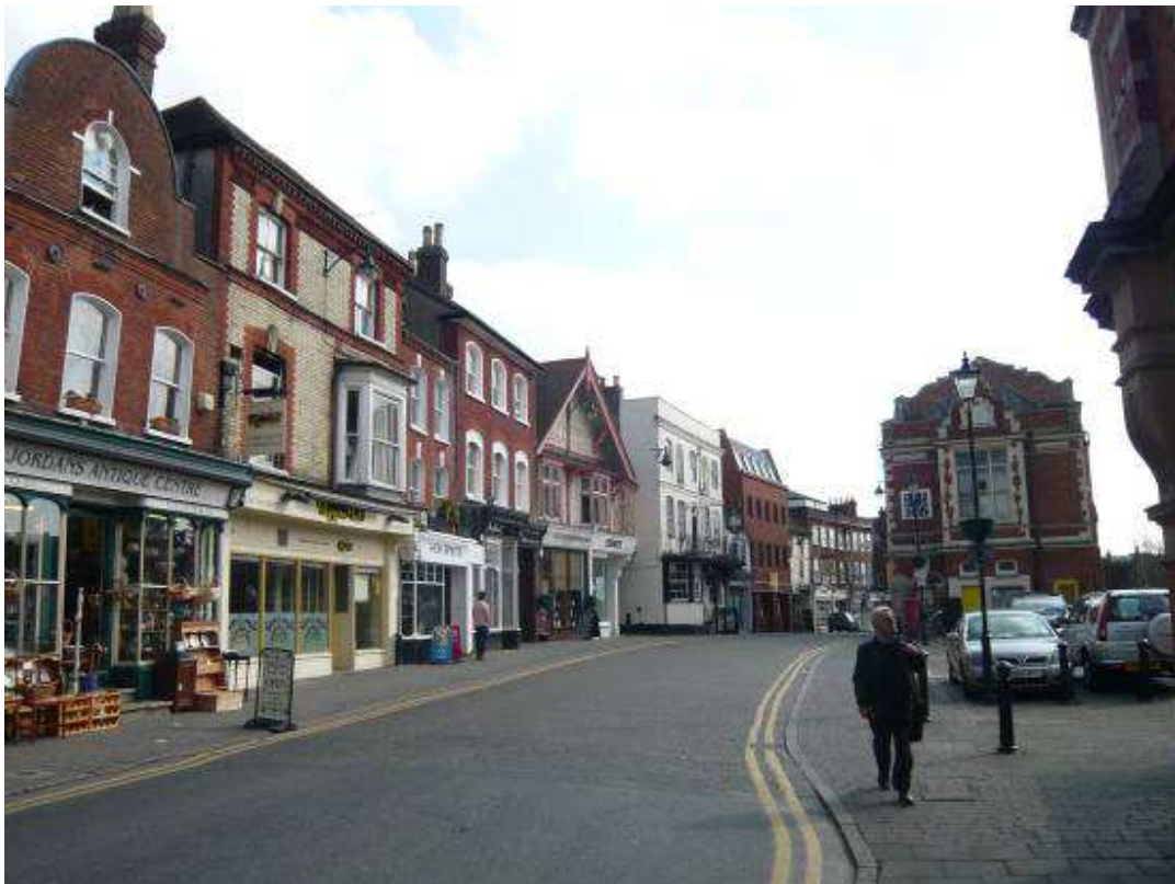
Figure 3: The curve of the High Street (here looking south) is an important part of the character of the street pattern
