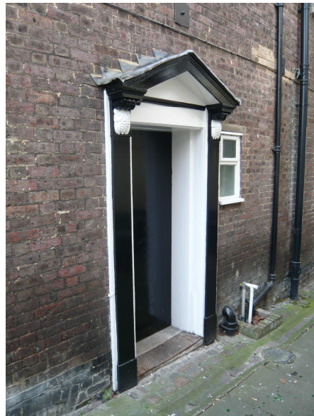
Figure 60: door surround and hood, High Street
