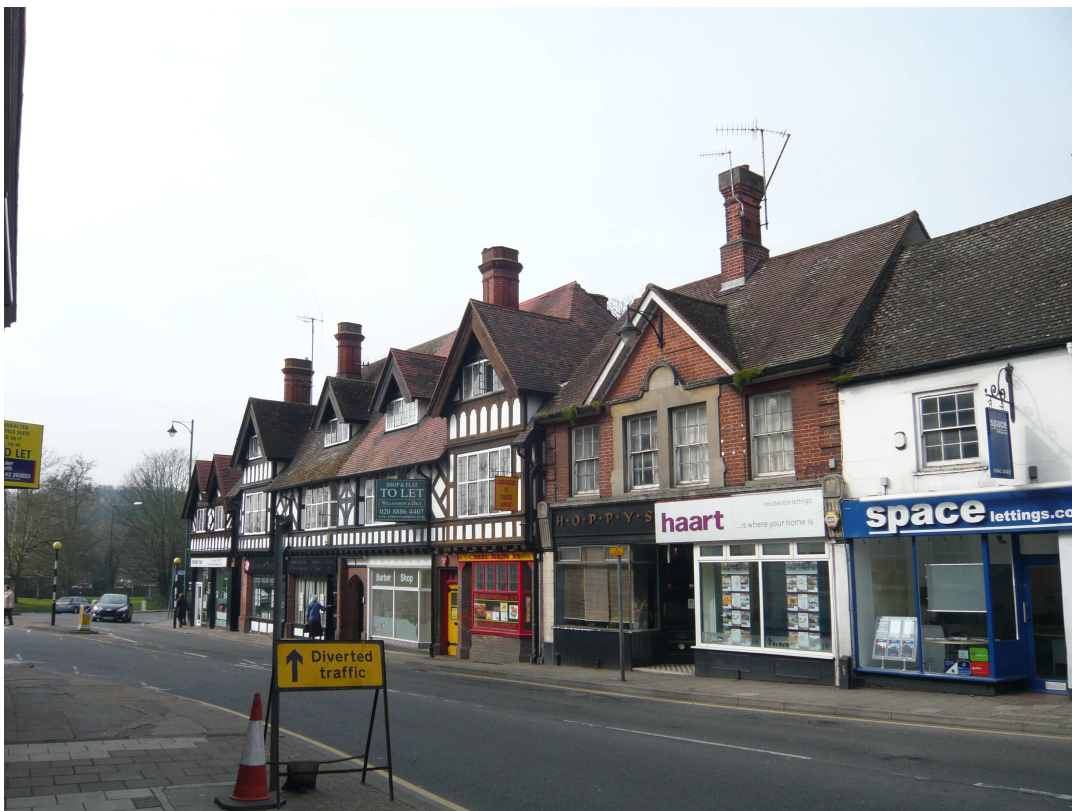
Figure 62: This group of Buildings to the north side of Queensway are of significant local architectural and historic importance
