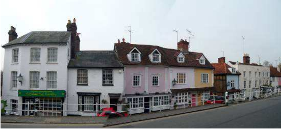
Figure 52: The consistent use of the multi-pane sash window unifies this part of the conservation area
