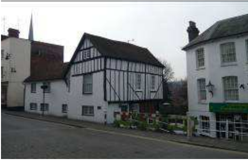
Figure 17: Timber-framed buildings seen adjacent to later rendered and brick buildings
