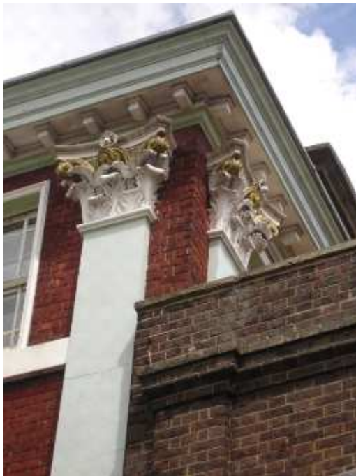
Figure 56: Corinthian pilasters to No.25 High Street
