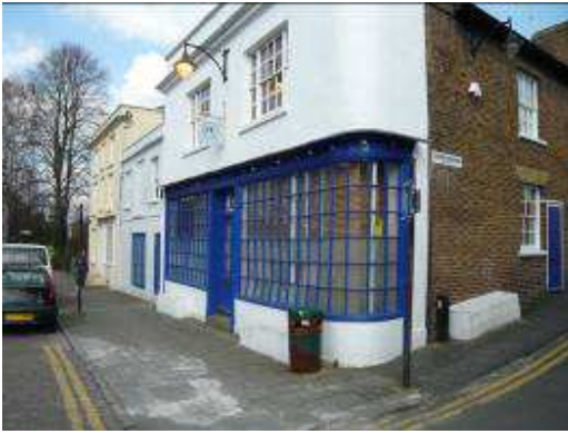
Figure 57: There is a good survival of traditional historic shopfronts
