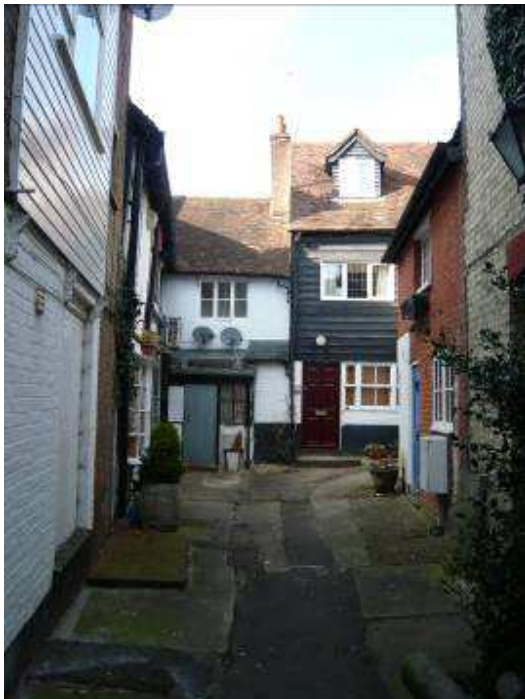
Figure 2: Development to the east of the High Street is often set in enclosed courtyards (rear of 71-73 High Street)
