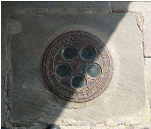
Figure 42: A early 20 th century cast iron inspection cover
