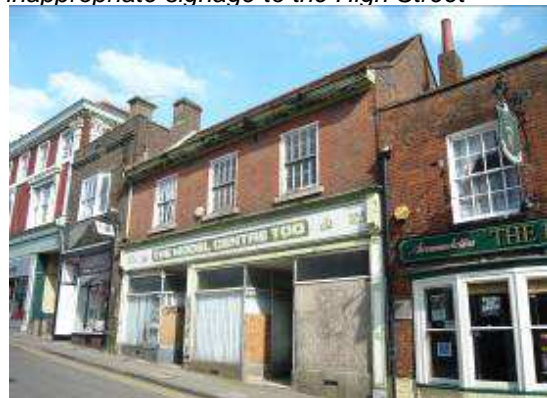
Figure 65: Nos. 21 and 21A a vulnerable building in poor condition requiring re-use
