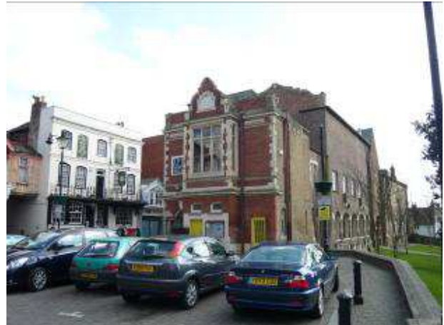
Figure 23: The Old Town Hall has a significant cultural as well as physical presence in the Old Town
