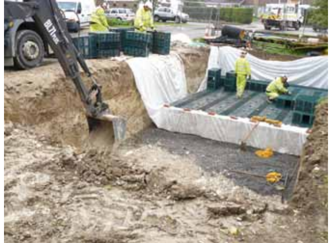
Improved drain maintenance to reduce flood risk
