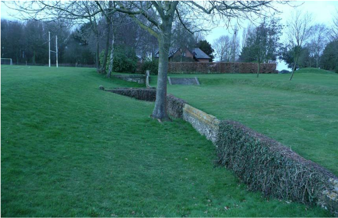
A surviving portion of the ha-ha and nineteenth century steps in the background
