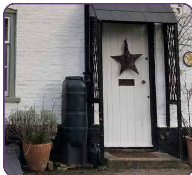
Figure 87: Water butts used for rainwater harvesting.
