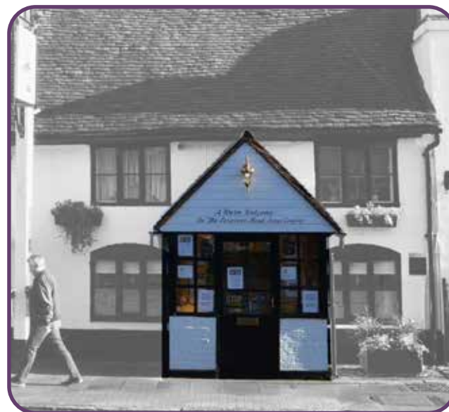
Figure 65: A protruding porch, High Street.
