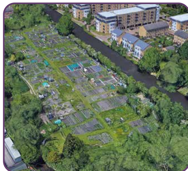
Figure 81: Aerial view showing the allotment by the canal in Inner Zone.
