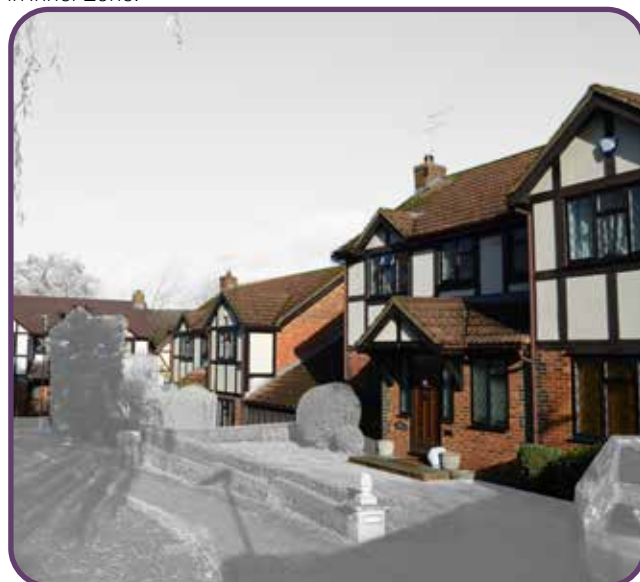
27 Figure 26: Timber-framed houses massing in the Peripheral Zone.
