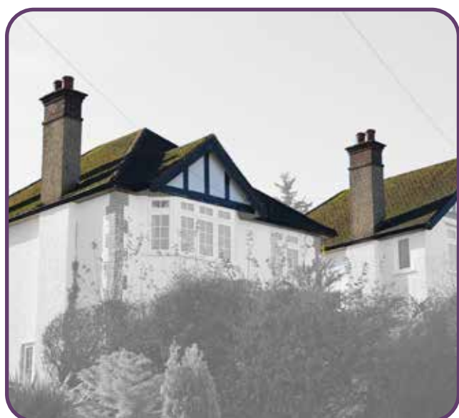
Figure 68: Hipped roof with slate in the Semi-rural Zone.
