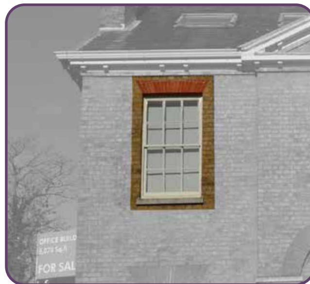
Figure 61: Multipane sash window in the Village Centre Zone..
