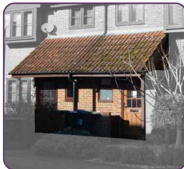
Figure 66: Wooden door with clay pantile roof in the Inner zone.
