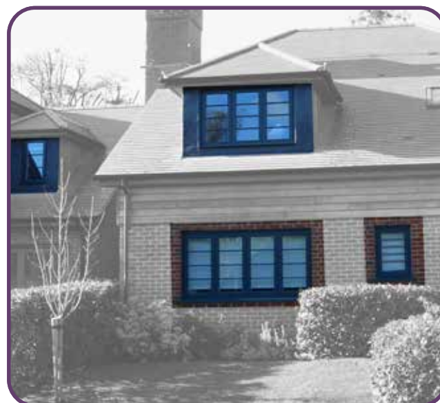
Figure 63: Casement window in the Semi-rural Zone.
