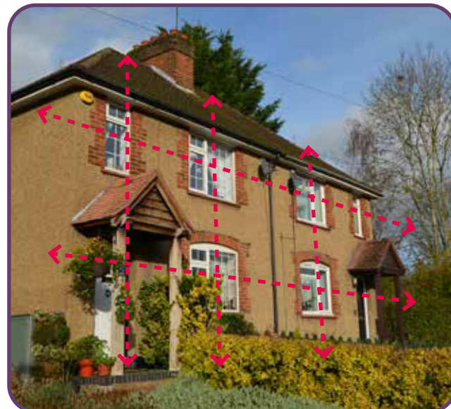
Figure 45: Windows spaced evenly along the building elevations in Rucklers lane..
