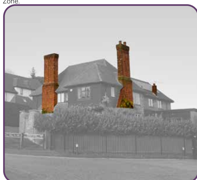
46 Figure 75: Tall chimney in the Semi-rural Zone.
