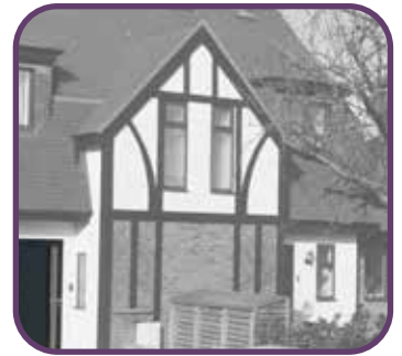
Mix of timber frame and red brick façade
