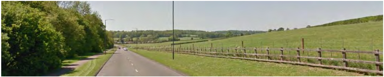
View from east end of Link Road towards Piccotts End, with Marchmont Farm site to the right.
