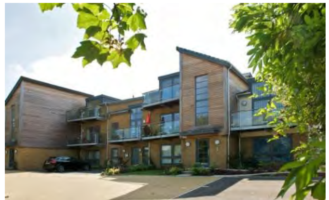
Figure 37: Although more modern in style than other examples the articulation of this facade provides opportunities for balconies with privacy from overlooking
