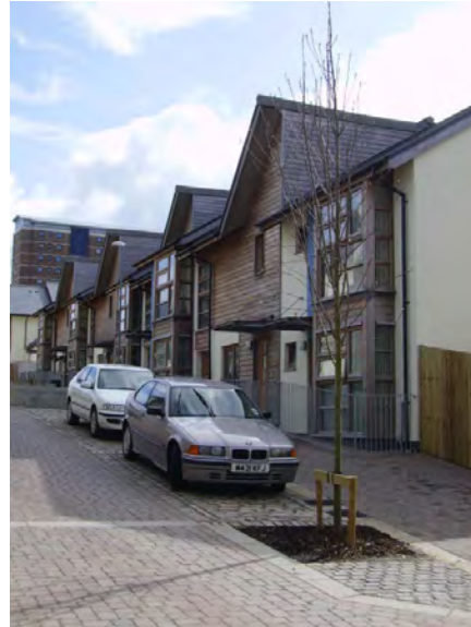
Figure 41: Well-designed on street parking can make a positive contribution to the street scene
