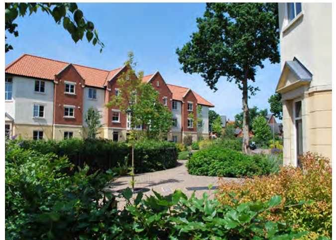
Figure 36: The articulation of the elevation of these flats help to break down its overall massing and is also in keeping with the surrounding housing development
