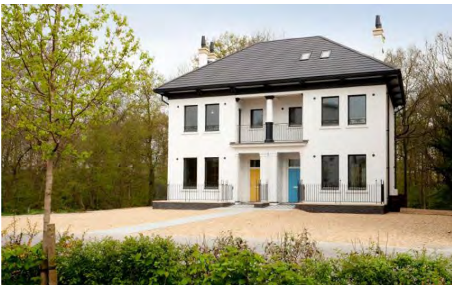
Figure 23: The Prince's Natural House at the BRE campus is a good example of the massing and proportions that would be appropriate for the Old Town site
