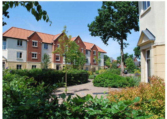
Fig 5.15 The articulation of the elevation of these flats help to break down its overall massing and is also in keeping with the surrounding housing development.
