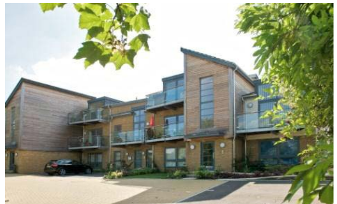
Fig 5.16 Although more modern in style than other examples the articulation of this facade provides opportunities for balconies with privacy from overlooking.
