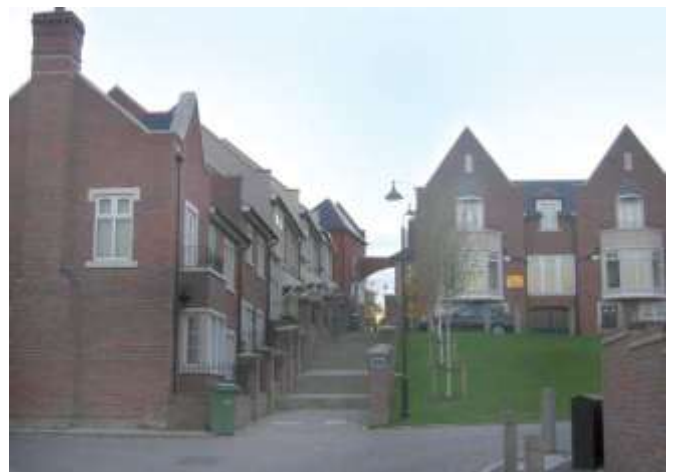
Fig 5.13 The buildings at Greenhithe step down a steep slope creating an interesting pattern of roofs, whilst also allowing level access to new homes.
