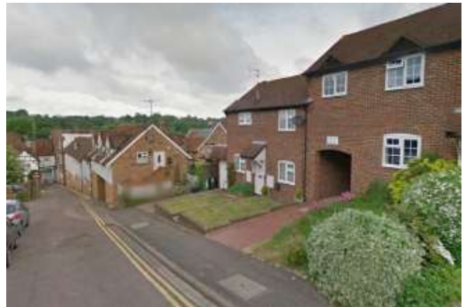
Fig 5.12 The existing homes on the nearby Chapel Street step down the steep hill and provide level access for each dwelling. Front gardens are terraced with the levels of the road.
