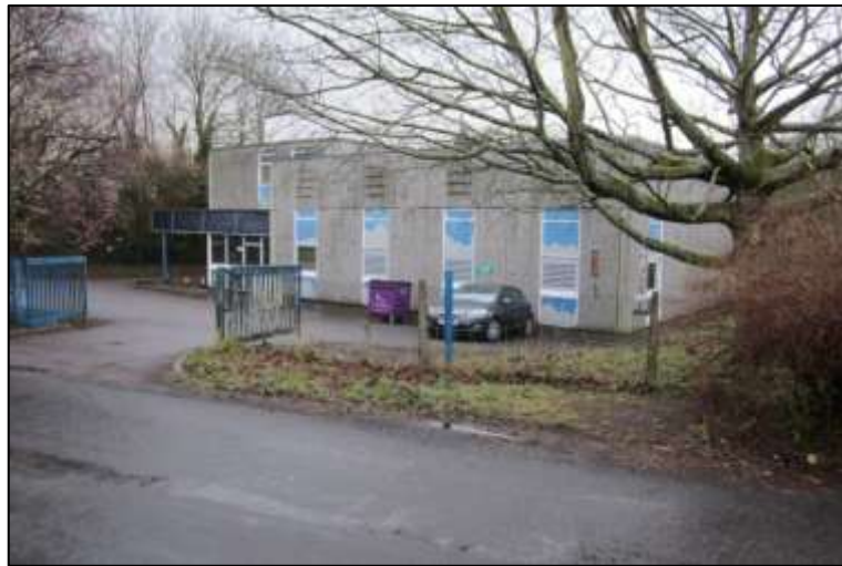
Plate 4: The telephone exchange
