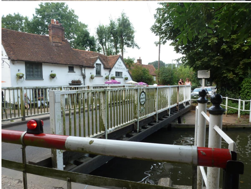
Figure 1 Pictures of swing bridge at Winkwell.
