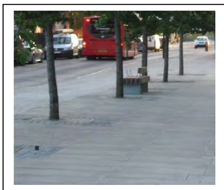
High quality concrete paving
