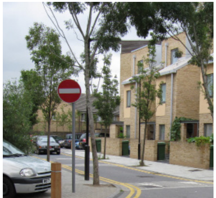
This example shows development at Harmony Place, London. Refuse storage has been integrated into front garden spaces. The design complements the architecture and screens bins from the street.
