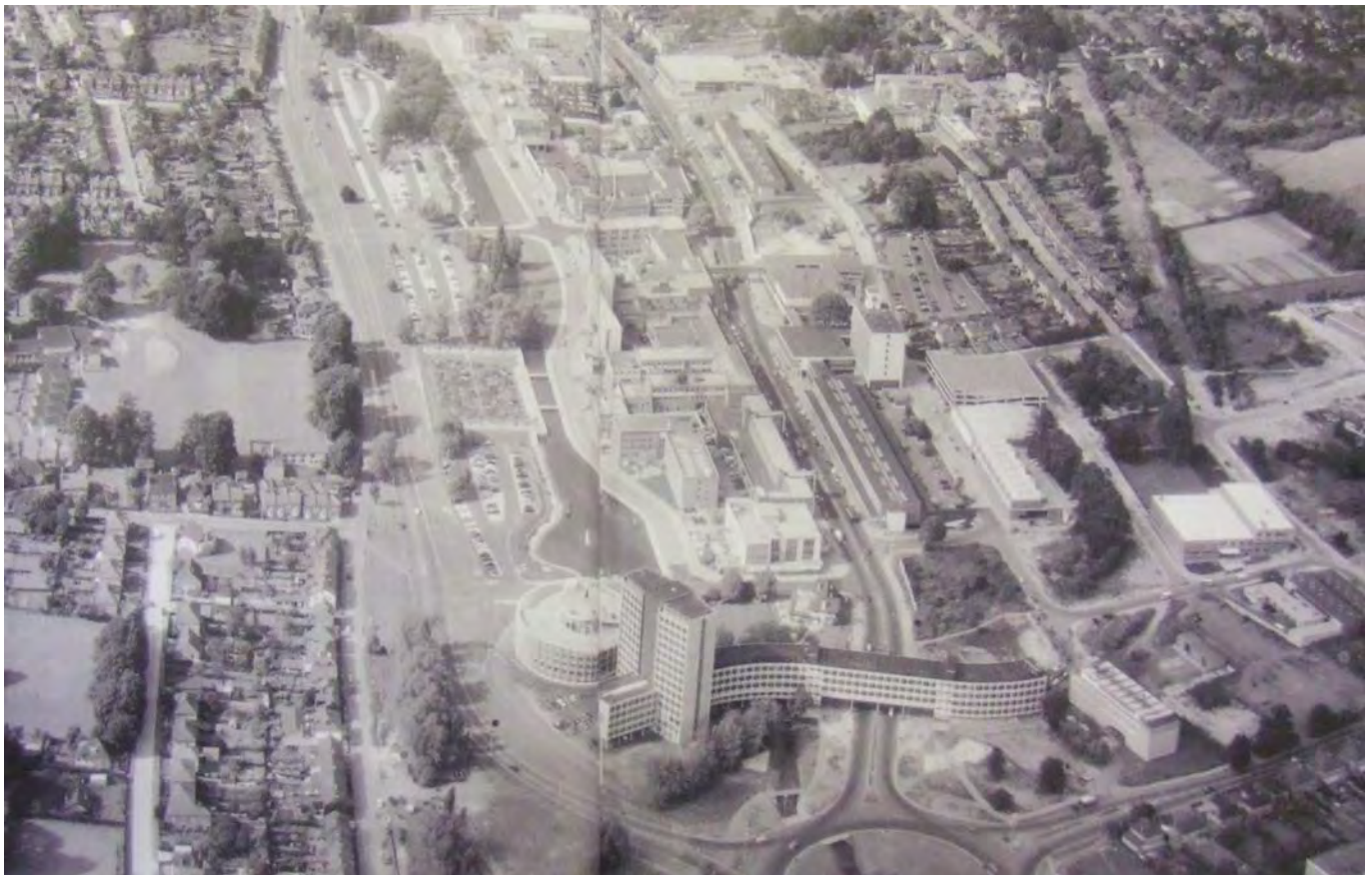
Figure A3.5 Completed New Town 1962
