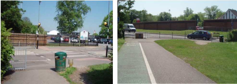
Figure 5 and 6 – Street furniture causing obstructions on Mortimer Hill, and worn grassed area at London Road.
