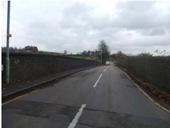
Figure 6 – Station Road Bridge
