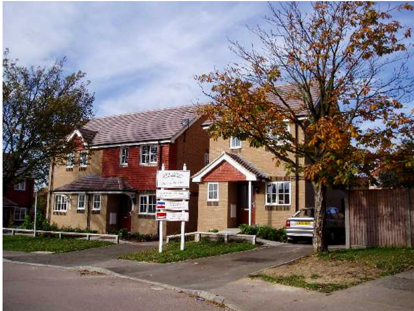
Recent development to the rear of 34-46 Deaconsfield Road
