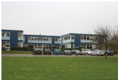
Existing school buildings
