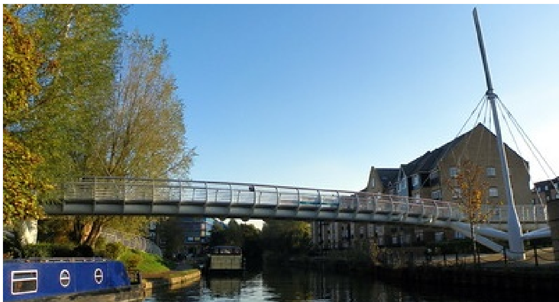
Figure 2-3: Apsley canal and cycle bridge
