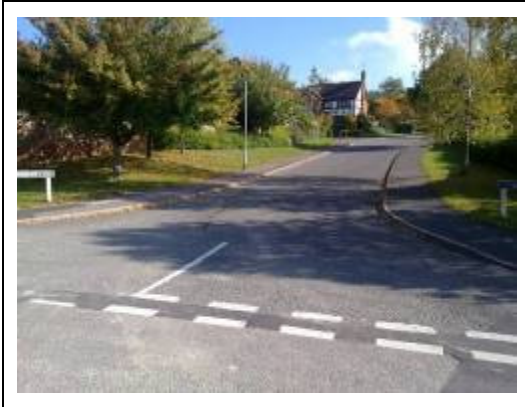
Plate 9 – eastbound view of St Katherine's Way
