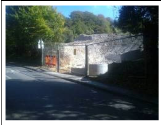
Plate 5 – northbound view of B4506 New Road adjacent to Tunnel Fields
