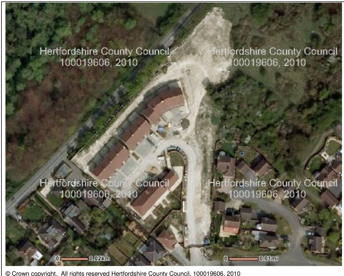
Figure 5 – Aerial View of Existing Site Layout
