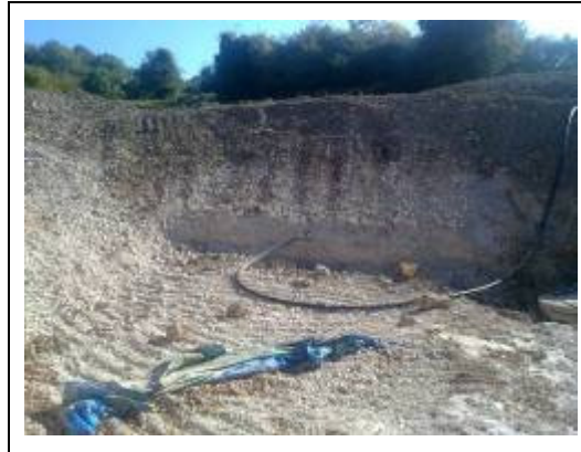
Plate 9 –level difference from New Road carriageway into Tunnel Fields site
