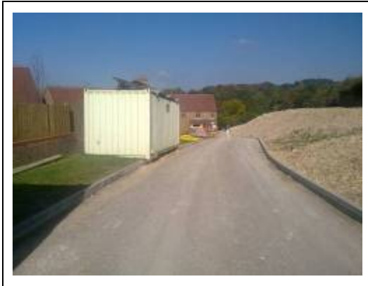
Plate 1 – northbound view of Tunnel Fields existing access road
