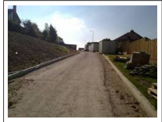
Plate 2 – southbound view of Tunnel Fields existing access road
